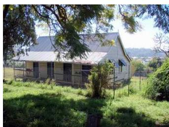
We moved on to the first house built by the Simmmons called *Beechwood*. This house was in poor repair, white ants having eaten through a lot of the woodwork. The verandahs were well rotted and by peeping in the side windows we could see the wooden panelled walls. The original cedar doors had been replaced or covered over. It was interesting to see the original stump work topped with tin plates, or ant caps, to prevent termites.
